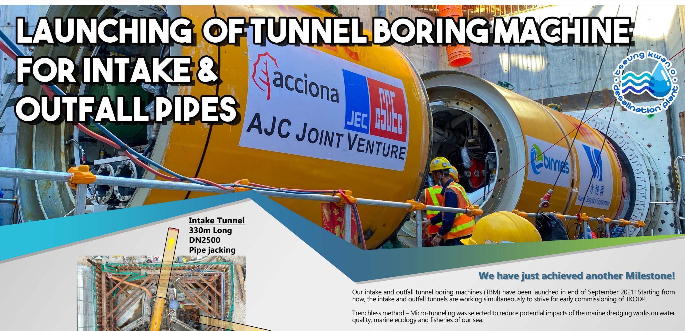
In addition to basic equipment in the TBMs for day-to-day excavation, such as cutter head, main drive, steering cylinder, slurry lines, grout lines and laser target, our TBMs have the following features to work under the submarine ground condition of the project.
